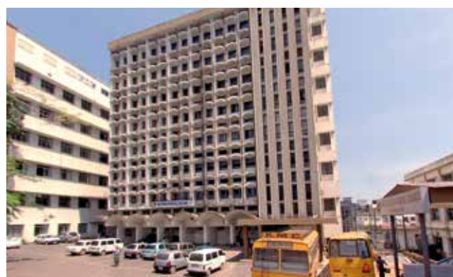
KMC Hospital Ambedkar Circle, Mangalore
